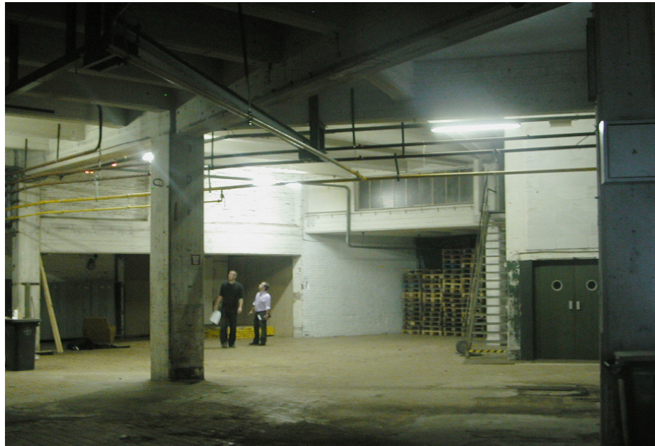
interior view, existing
