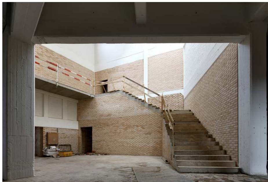
interior view, during renovation
