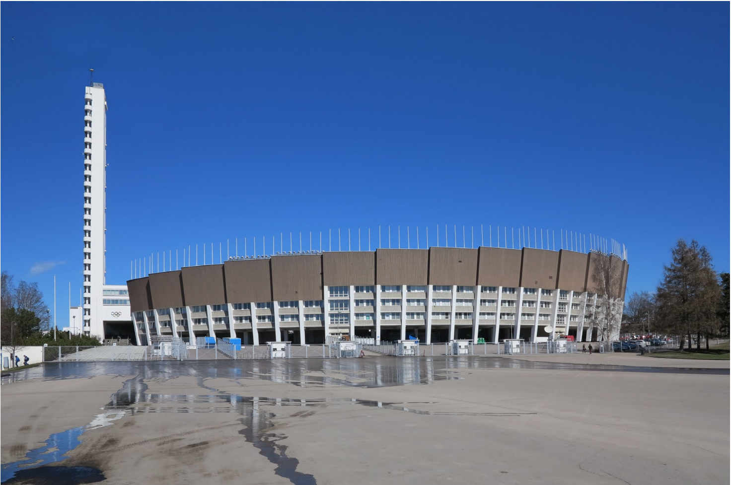
2013 The south facade of the stadium before the refurbishment. The timber cladding, brick work, windows and doors were badly eroded.
