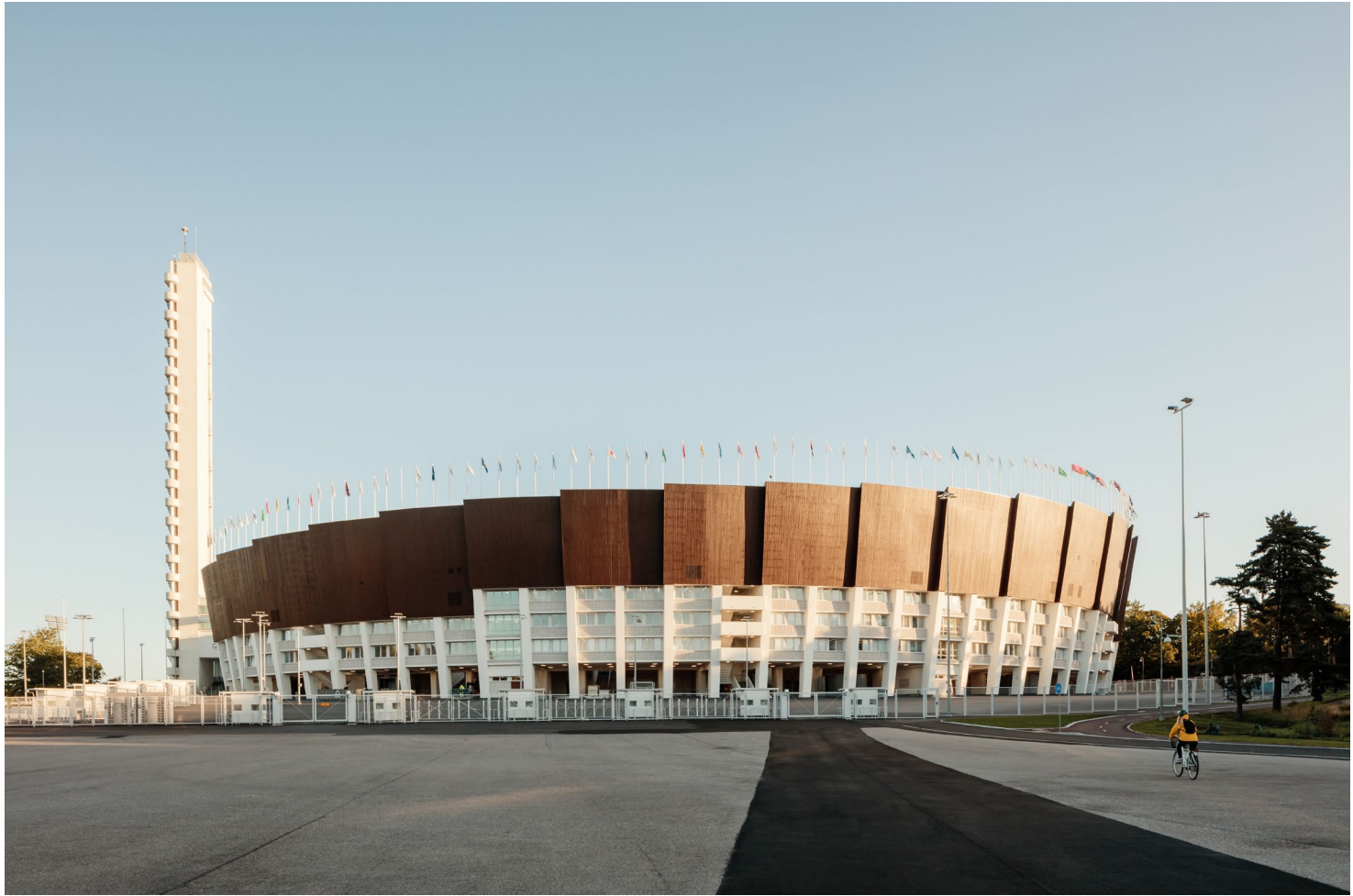
2020 The south facade of Helsinki Olympic Stadium after the refurbishment. The facade line was raised by a couple of meters to conceal the new canopy and to preserve the iconic external form. (Photograph: Tuomas Uusheimo)
