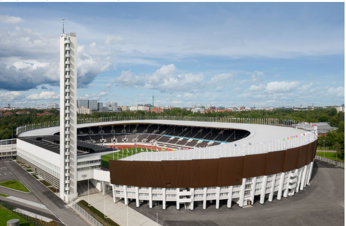
2020 The Stadium after the refurbishment. The eastern canopy was extended and now covers most of the spectator seats. (Photograph: Wellu Hämäläinen)
