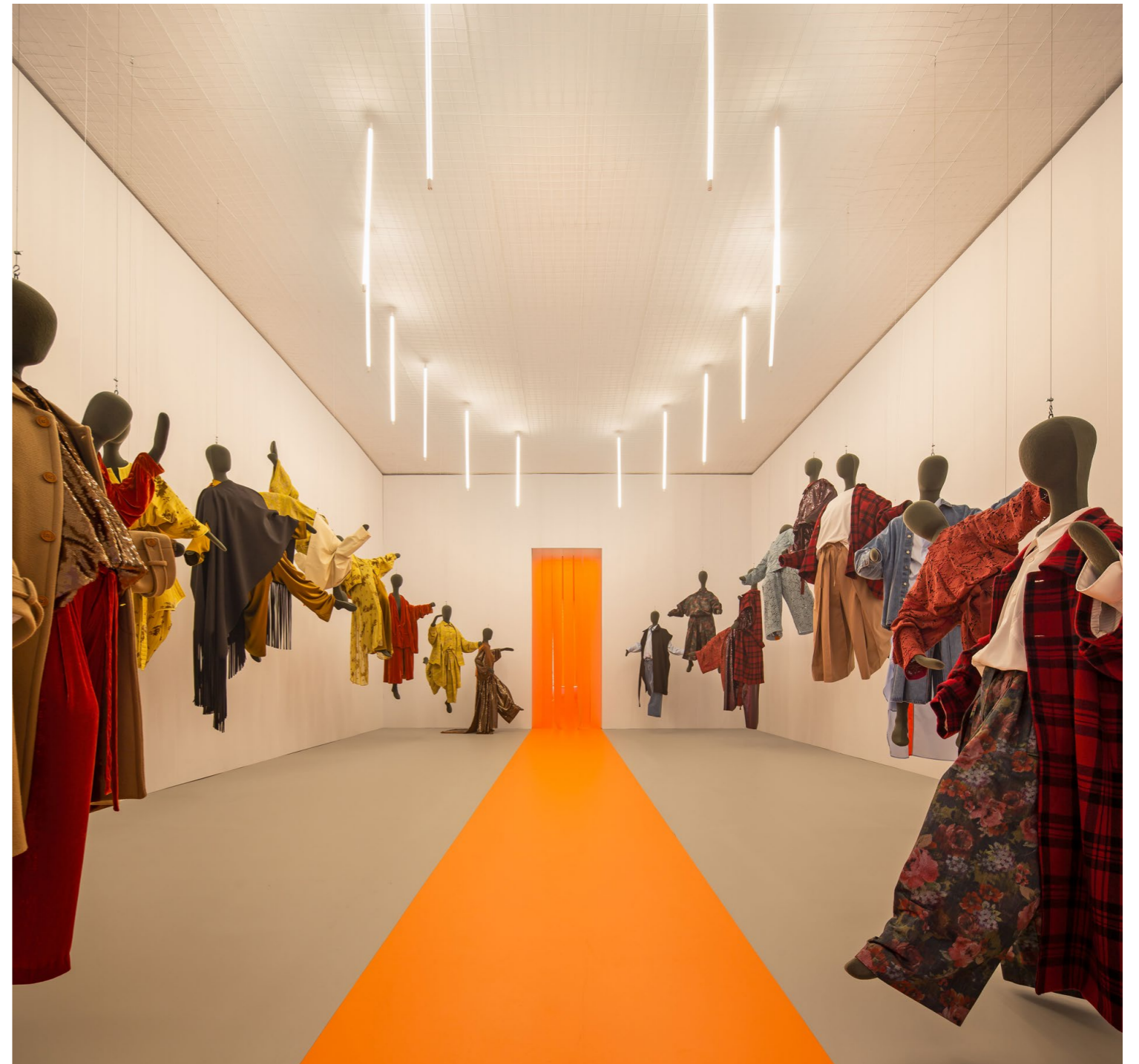
The ceiling is made by a simple and thin fabric grid, to avoid the use of heavy or non-recyclable materials. Some weight testing were needed before lifting up the solution.
