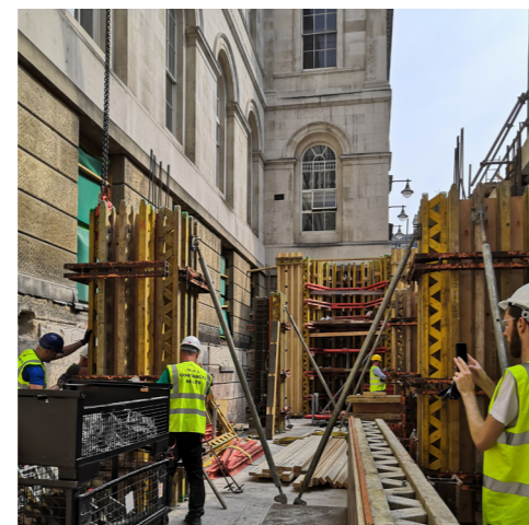
Forming the concrete lightwell structures
