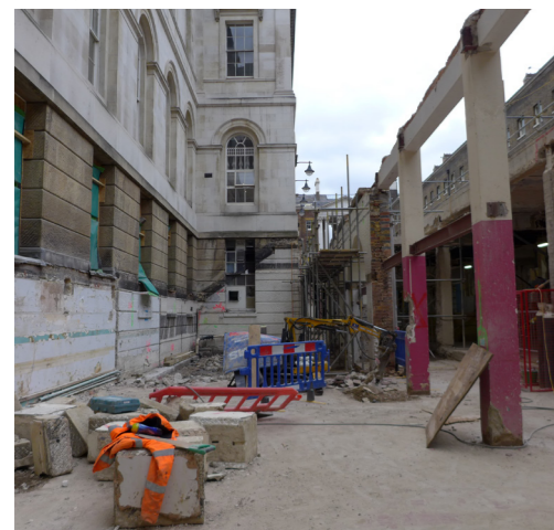
During construction - demolition of existing lightwells
