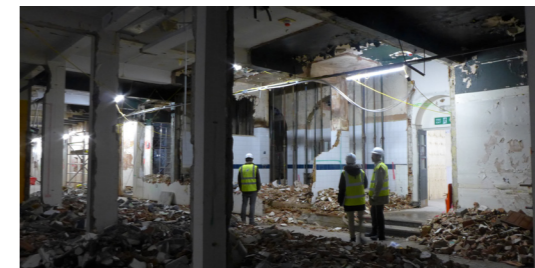
Arches were concealed and covered in plaster and tiling.
