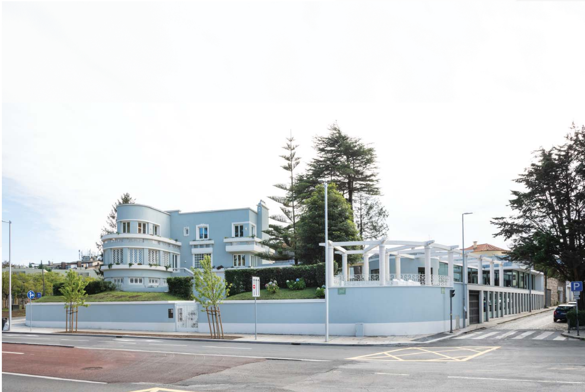
The rehabilitated house and new extension viewed from Avenida da Boavista (2024)
