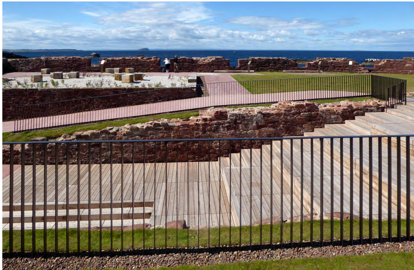
Finished view of performance space, coastal garden, existing stone walls and the distant horizon
