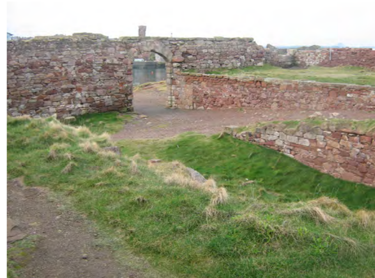
Previous condition - walls of former hospital building
