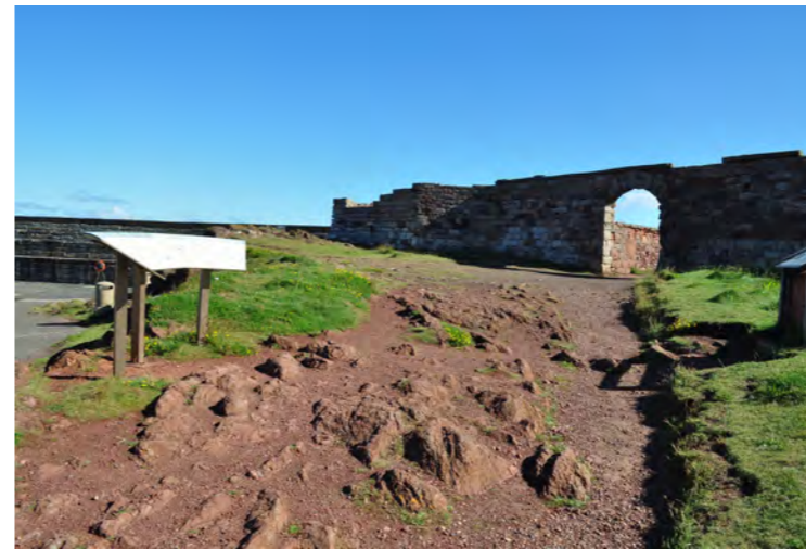
Previous condition - access path, uneven and inaccessible
