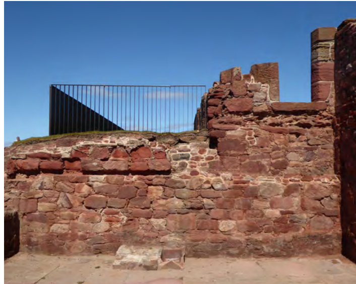
Composition of existing walls and contemporary railings
