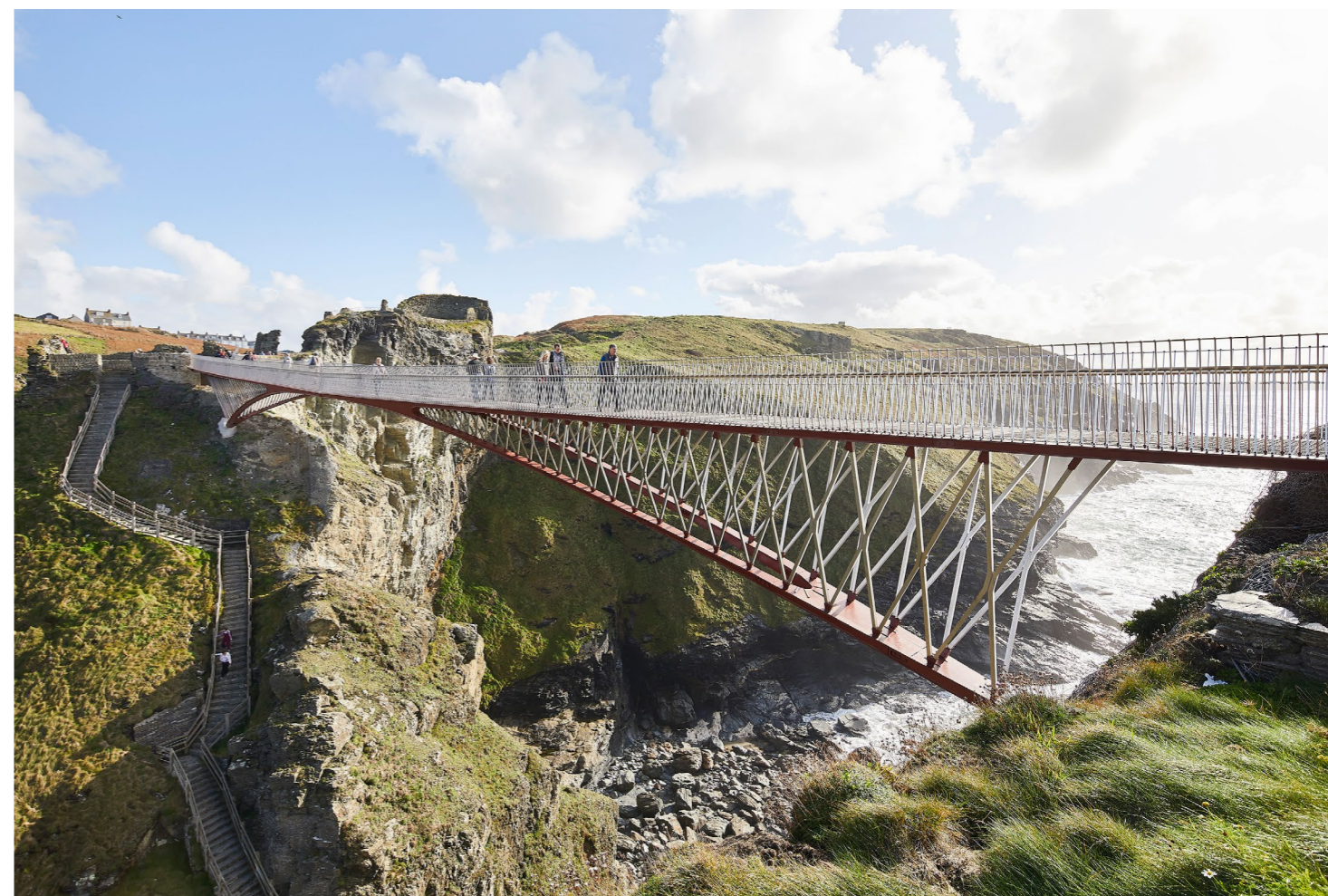
TINTAGEL FOOTBRIDGE, CORNWALL UK - Ney & Partners and William Matthews Associates - CATEGORY B
