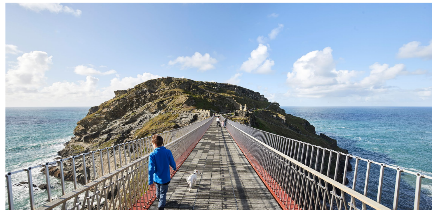
TINTAGEL FOOTBRIDGE, CORNWALL UK - Ney & Partners and William Matthews Associates - CATEGORY B
