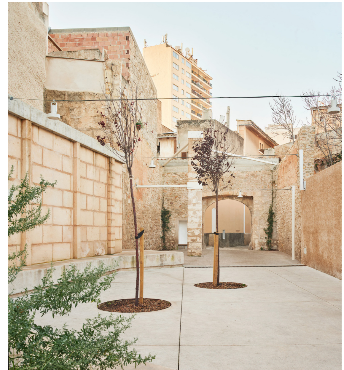
Concrete pavement with a very high proportion of 15/25mm aggregate (aggregate incorporated into the surface)
