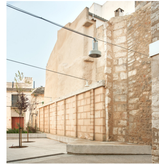
Deactivated concrete pavement with quartz and graded corundum aggregate 3/5mm.
