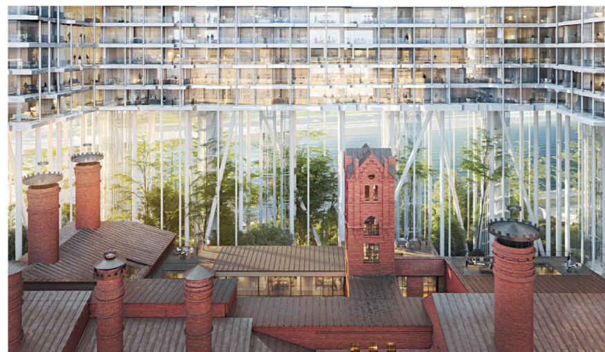
Picturesque silhouette of Building 3 is a strong element defining the identity of the site. Four new light-wells, together with a courtyard, bring daylight into the deep floors and emphasize the original vertical cluster structure of the building, without interfering with the historical façade.
