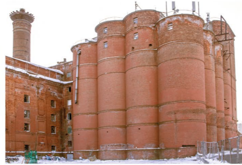
Silos on west end of Building 3
