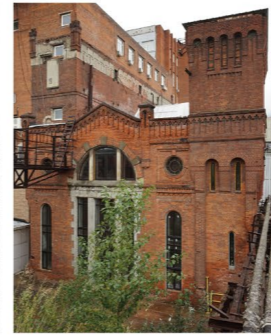
Remaining part of Building 2
