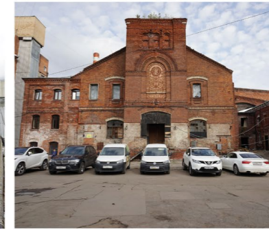
South facade of Building 1 - Western part
