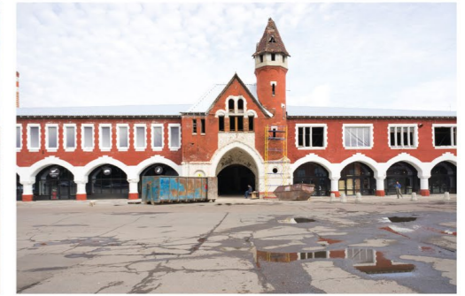
South facade of Building 1 - Eastern part
